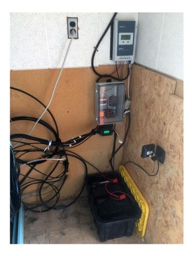
The solar charge controller was changed from a PWM (Pulse Width Modulation) to a MPPT (Maximum Power Point Tracking). The new controller is a EPevers Tracer 3210AN with a RS-485 status port and battery temperature probe.
